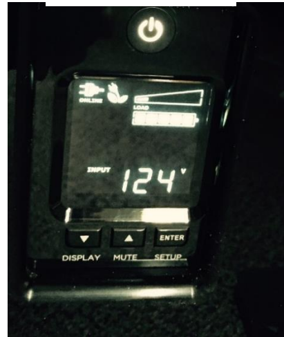
UPS Control Panel
